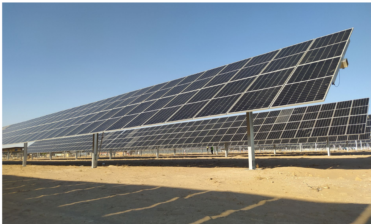
Figure 14. Solar panel installation
