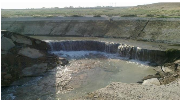
Photo. 18. Failure on the TM-2 canal (left) and blowout in the GPS-1 pressure pipeline.
