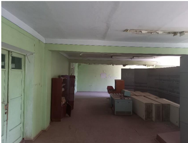
Photo. 17. Dysfunctional automated water distribution control desk on the TM-1 and TM-2 canals of the Zafarabad SRIA.
