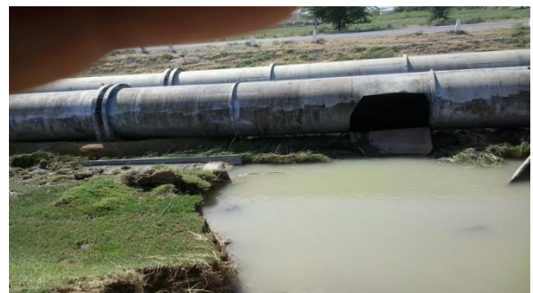
Photo. 18. Failure on the TM-2 canal (left) and blowout in the GPS-1 pressure pipeline.
