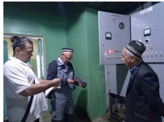
Photo: Measurements of water and electricity consumption in the pumping station Golodnaya Stepskaya Pumping Station - 1 with the support of Grundfos
