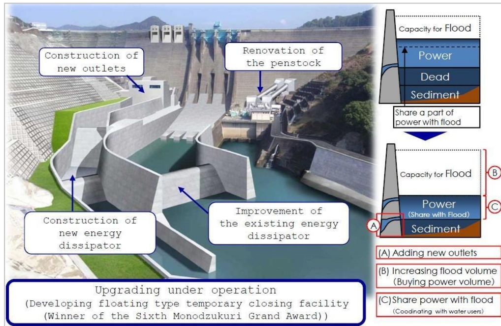
Figure 5-16 Upgrading of Tsuruda dam (Courtesy of Water and Disaster Management Bureau, Ministry of Land, Infrastructure, Transport and Tourism, Japan)
