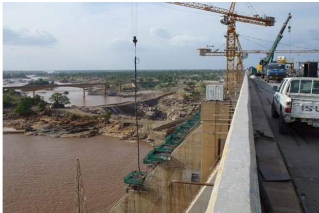
Figure 5-20 Heightening of Roseires dam ( http://pf.bbrnetwork.com/ )
