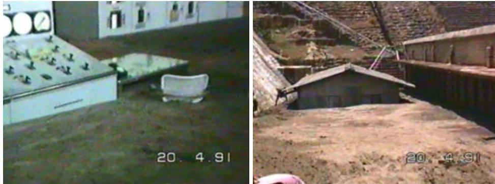
Figure 3-20 Sediment deposited in (left) and around the powerhouse (right) as a result of a sediment hazard during flushing operation at Pillur reservoir in India (Giri et al., 2019)
