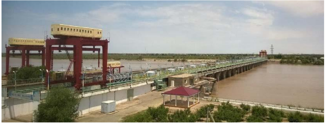
Figure 2-3 Takhiatash hydrostructure, located downstream of Tuyamuyun, in Karakalpakstan (UzNCID, 2020)
