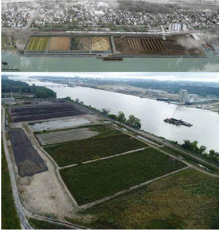
Figure 3-30 Various cells for the placement of dredged materials
